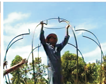
19- place ring at top of frames
