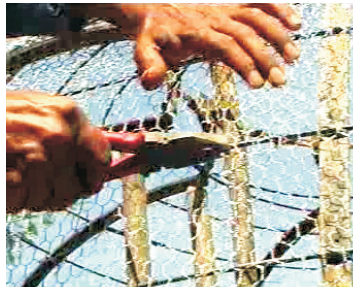
24- Fix chicken mesh to frames
