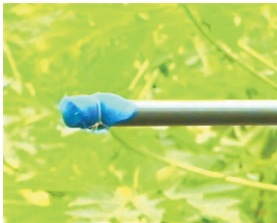
50- Tie net on overflow pipe
