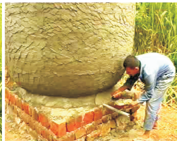
30- Place cement at base
