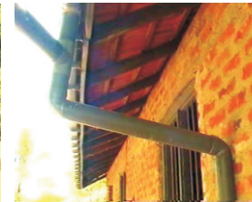
52- Install run-off pipe
