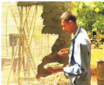
28- Place first layer of cement
