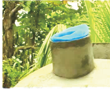
48- place bucket on tank
