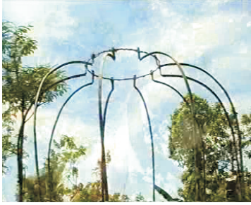
20- Tie ring to top of frames
