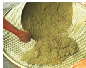
42- Lay cement on mesh
