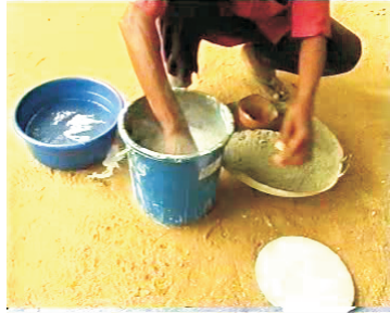
38- Prepare waterproof slurry
