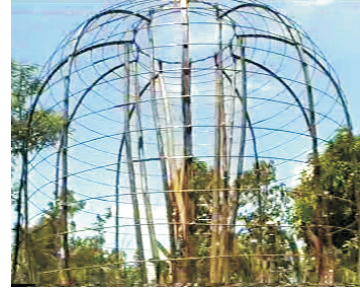
22- Place props inside framework
