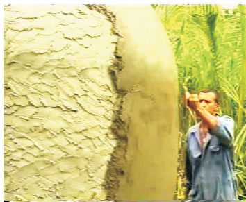
29- Place second layer of cement
