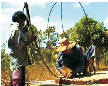
17- Fix the metal frames
