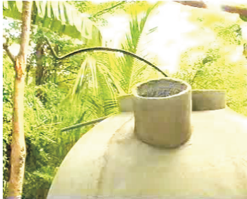
37- Take frames outside tank
