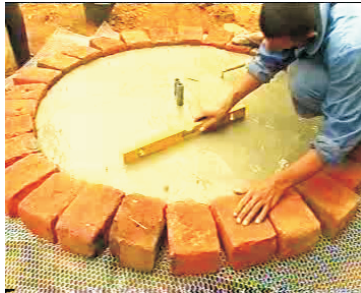
15- smoothen concrete surface
