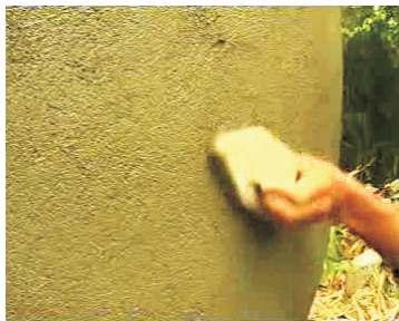
31- Smoothen outer surface
