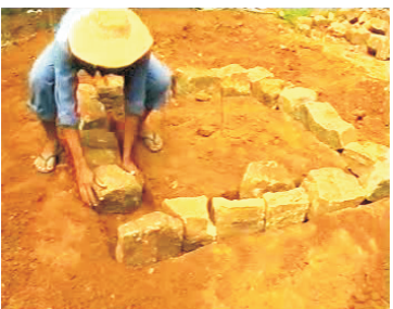
4- Cement the stone foundation
