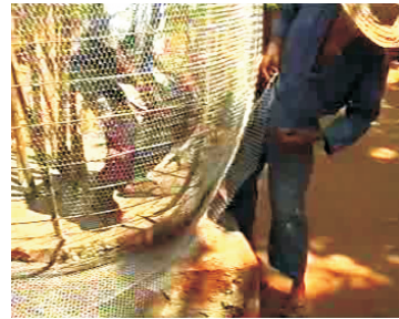
25- Fix base layers of mesh
