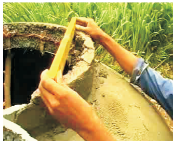
32- Smoothen lip of tank
