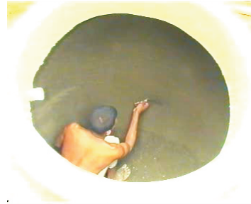
39- Smoothen inside with slurry
