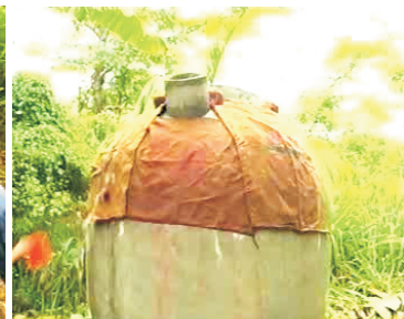
33- Allow tank to cure
