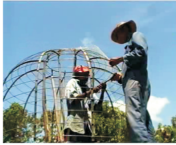
21- Fix metal hoops to frames
