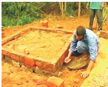
5- Cement the brick layer
