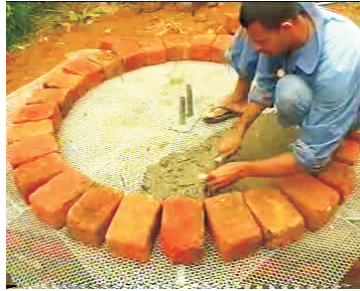
14- Lay concrete within brick circle
