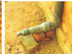
53- Fix stopper to runoff pipe
