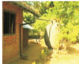
51- Install rain water pipes
