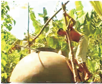
34- Erect scaffolding - enter tank
