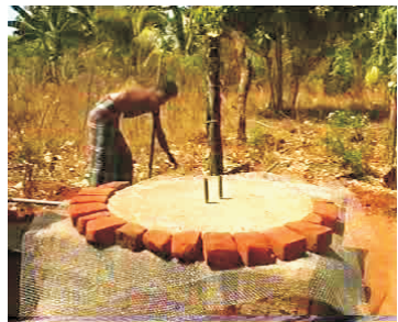
16- Remove row of bricks
