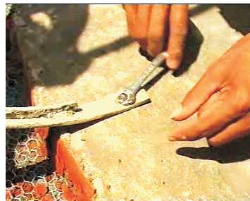
18- Tighten nuts at frames
