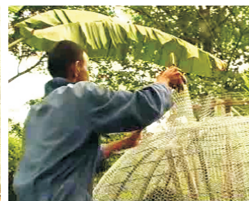
27- place mesh cylinder on tank
